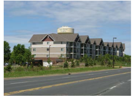
Inver Grove Heights Water Tower
