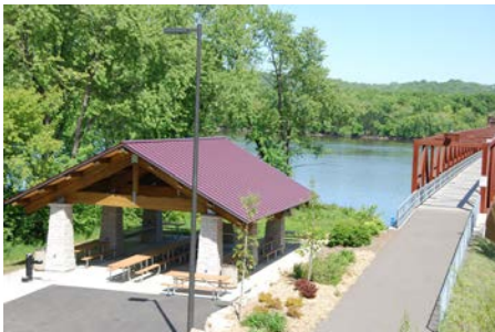
Swing Bridge Park
