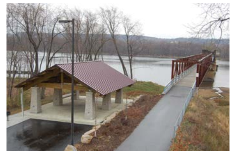
Swing Bridge Park
